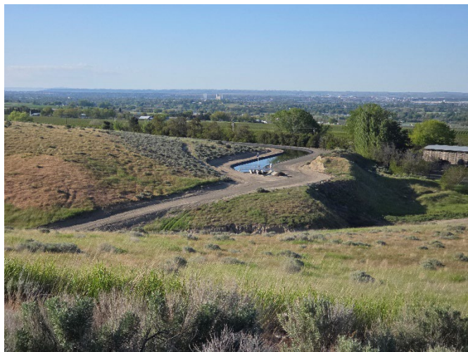
Kennewick Irrigation District canal facility in Finley
